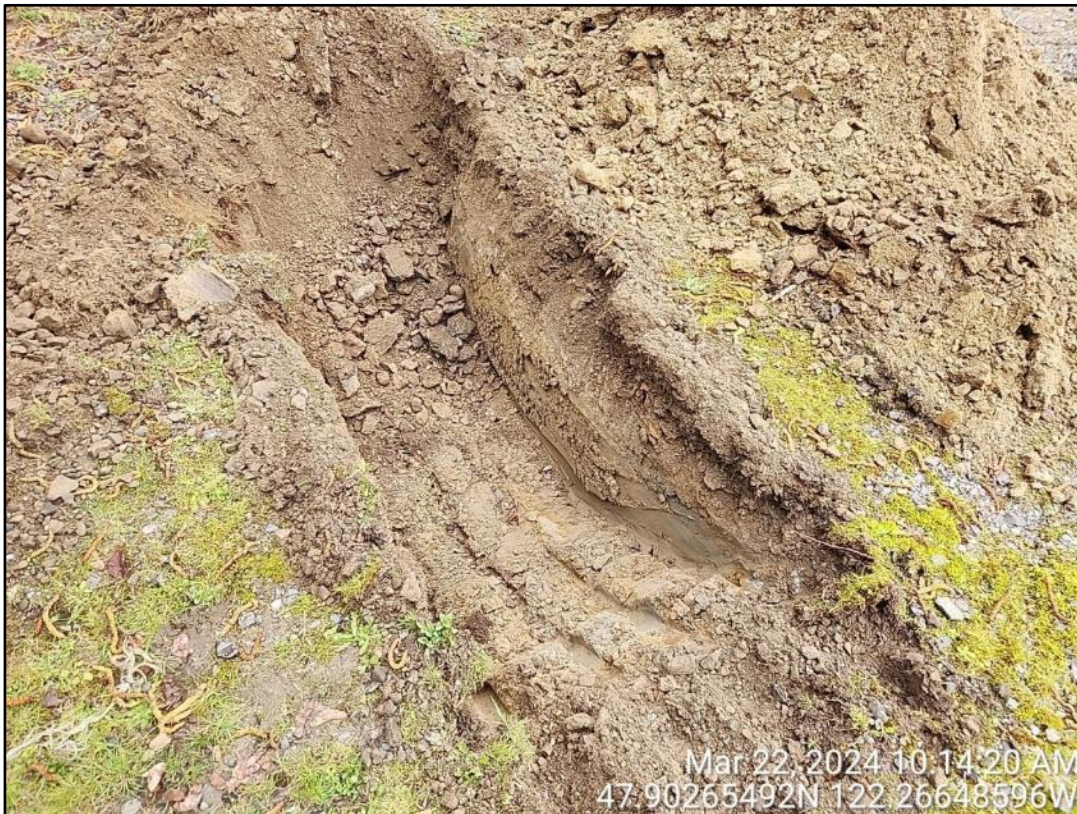
Image of TP-1 excavated to 3 feet below ground surface (bgs).
