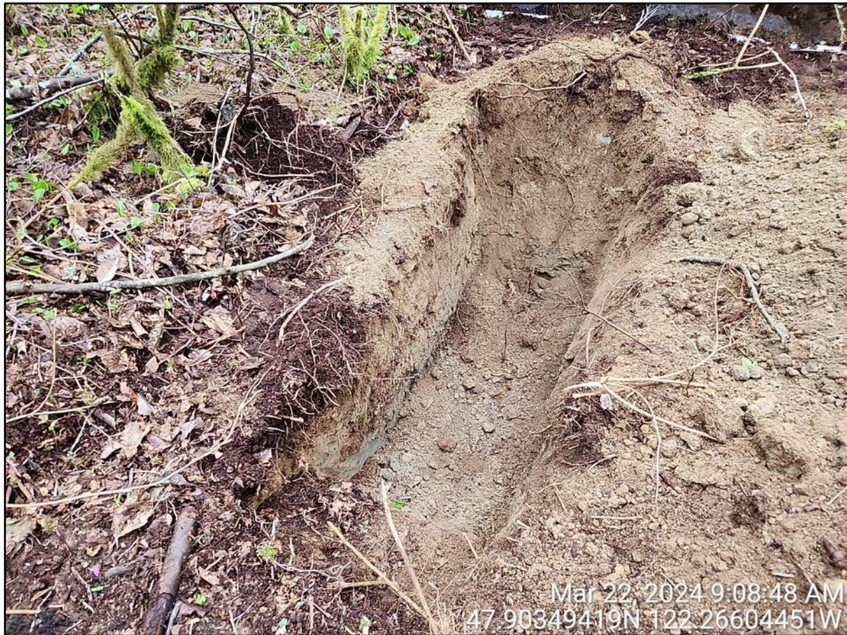
Image of TP-5 excavated to 3 feet below ground surface (bgs). Groundwater was not encountered at time of exploration.
