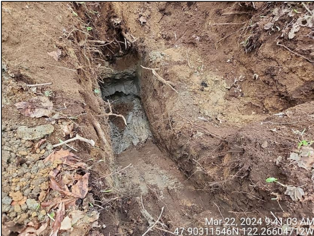
Image of TP-6 excavated to 8 feet below ground surface (bgs).
