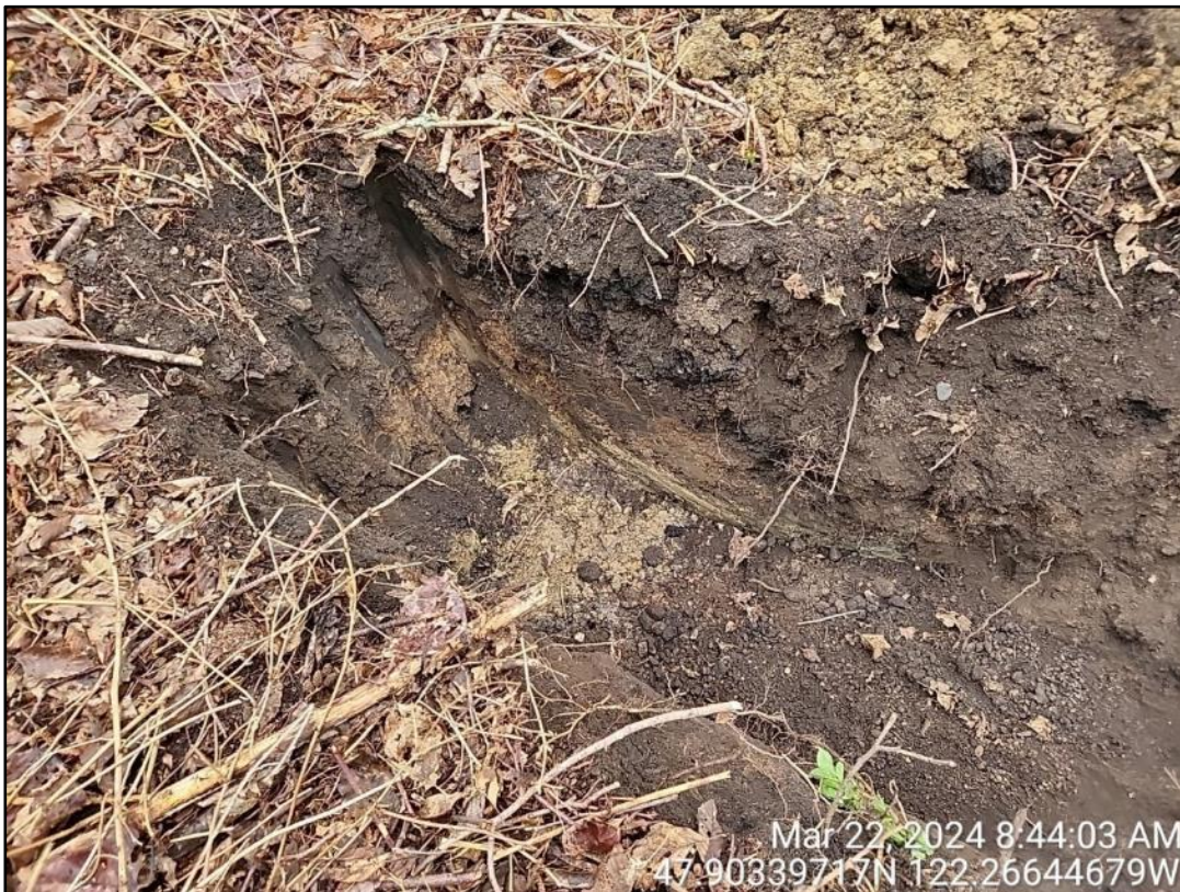
Image of TP-3 excavated to 4 feet below ground surface (bgs).
